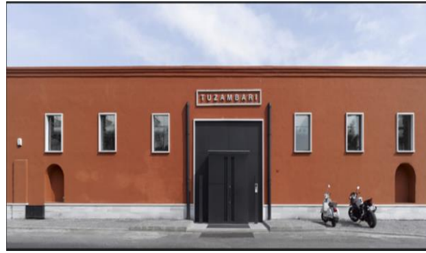
Figure 1. DDB Salt Warehouse entrance elevation (URL-1)
